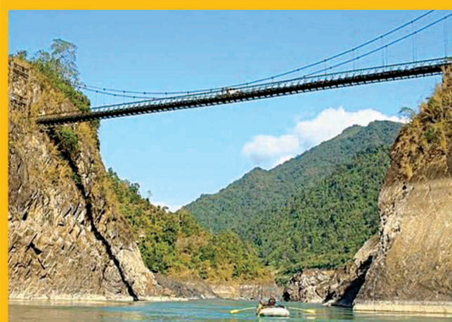
360 Ft Suspension type Bridge on Siyom River at Paksing, Arunachal Pradesh, India
