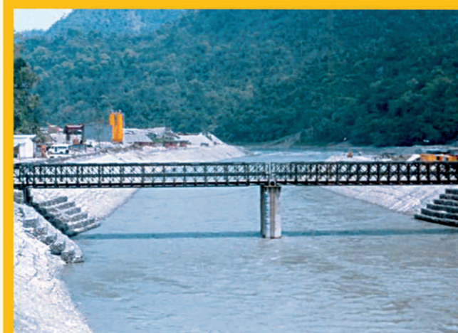
Multi-span Bridge (120 Ft & 130 Ft) on river Teesta in West Bengal, India
